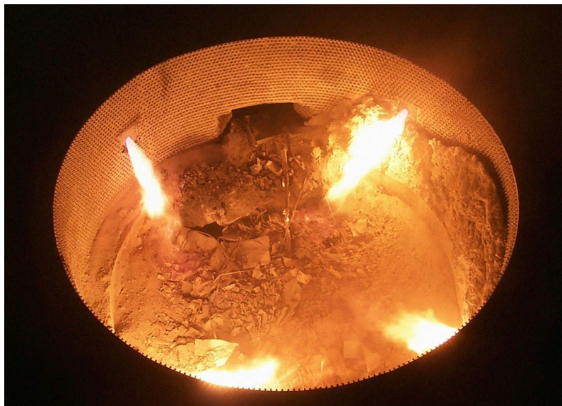
Fig.1 - Four CoJet injectors in operation in an EAF at the Nucor Berkeley plant, USA.
