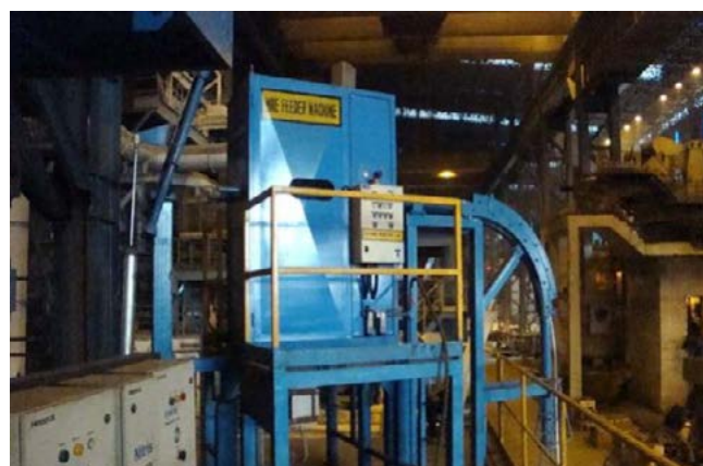
Fig.15 - New wire additions in LF.
