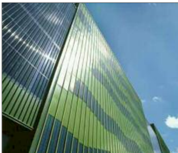
FIG. 7 Facade with building integrated photovoltaic elements.
